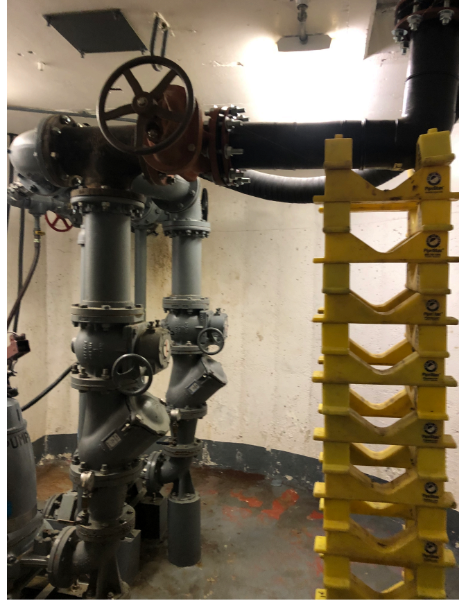
Photo 2: Lower level showing temporary piping (temporary discharge) and supports.
