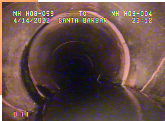
▲ Protruding lateral must be ground flush with pipe wall prior to rehabilitation to avoid tearing the liner and creating a bulge in the final end product.
