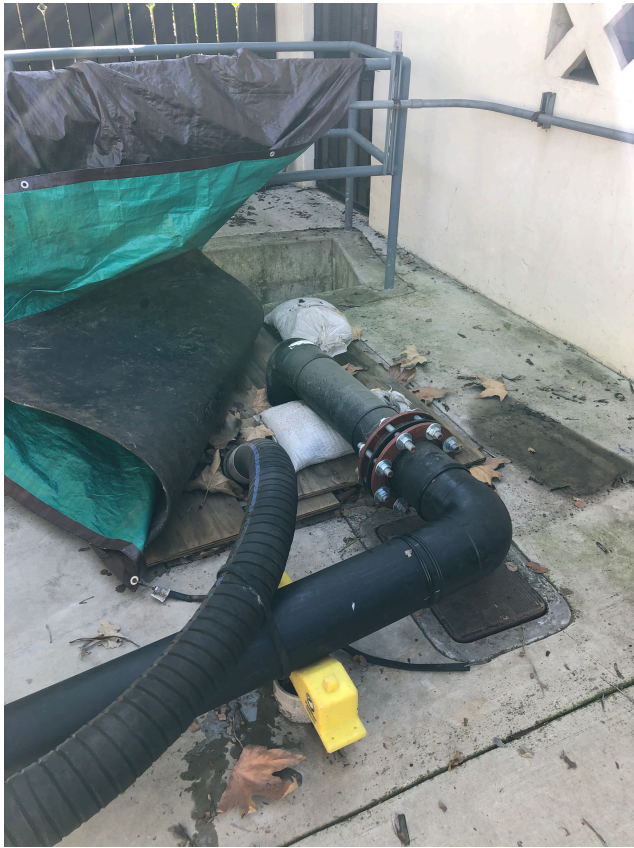
Photo 5: Top level showing temporary piping exiting shaft of dry well.
