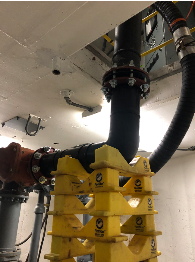
Photo 3: Lower level showing temporary piping through dry well shaft and supports.
