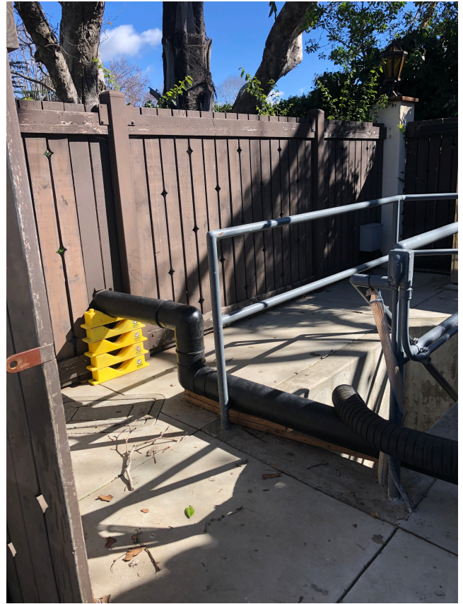
Photo 6: Top level showing temporary piping and supports above grade through fence.
